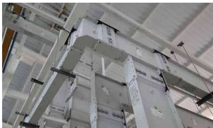
Example of Legrand busbar system
