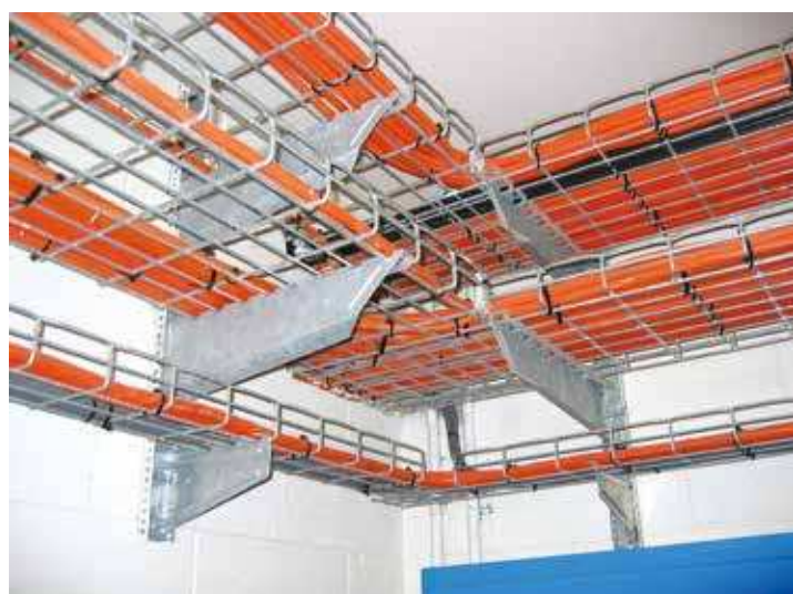
Example of space used by cable tray system
