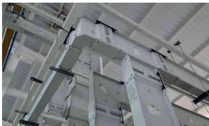
Example of Legrand busbar system
