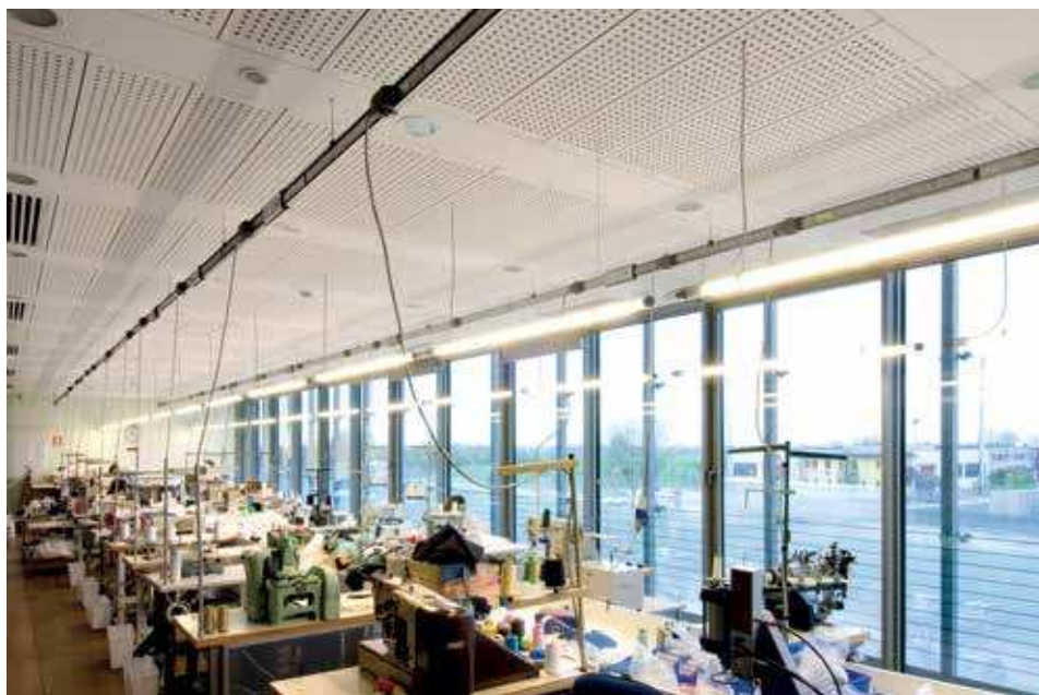
Example of lighting and small power distribution
